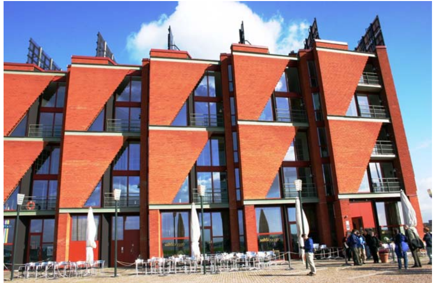
Seattle based participants on an Urban Sustainability tour of Western Harbor looking at the vertically mounted solar collectors atop this restaurant and commercial building. (photo by Mark Brumbaugh, Brumbaugh & Associates)
