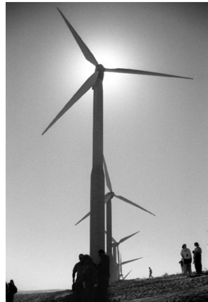
The Stateline wind project, on the border between Washington and Oregon, was when constructed one of the largest wind farms in the world. (Photo courtesy of Renewable Northwest Project)
